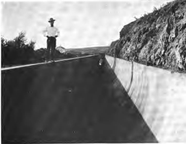
FIG. 80.—Semicircular Concrete-lined Section of Main Canal, Umatilla Valley, Oregon.
